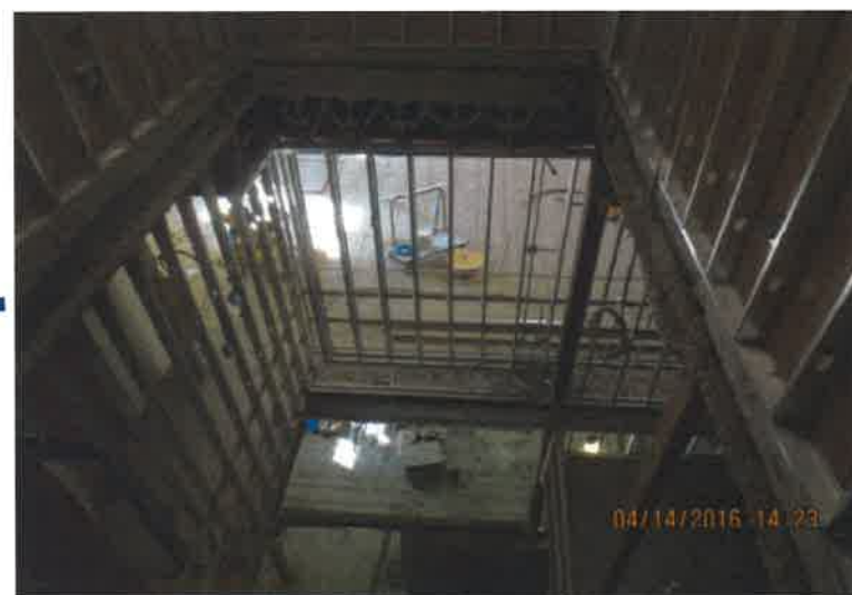
Framing & Decking For Main Stair
